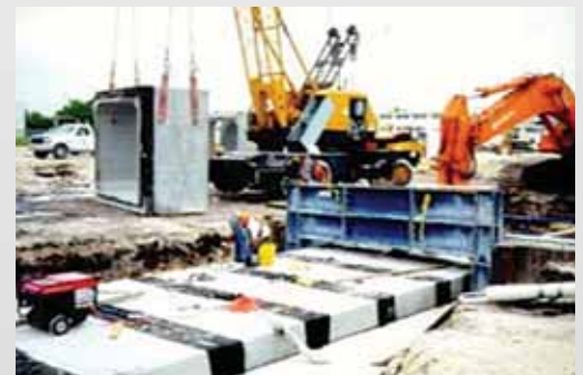
BOX CULVERT INSTALLATION WITH 18' HIGH X 18' WIDE CLEARANCES
