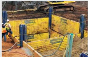
Remediation Slide Rail
