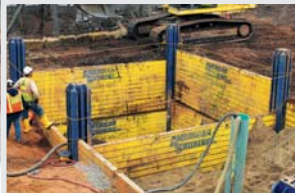
Remediation Slide Rail
