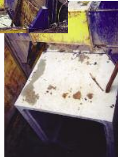
Above: installation of a 23'D x 12'H x 10'W precast concrete box culvert using Mega Rolling Strut Slide Rail with a clearance of 16' under the cross brace for the NYCDEP in Brooklyn, NY.
