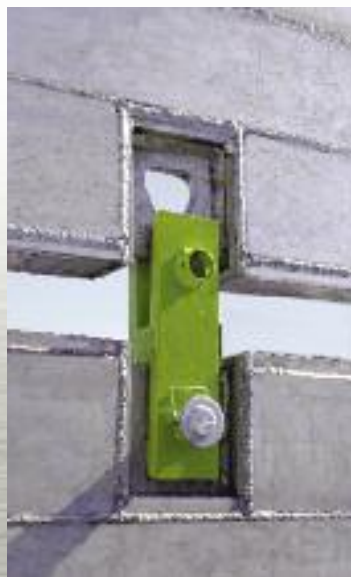
"H" BRACKET EXTENSION CONNECTORS WITH INSIDE KEEPERS
