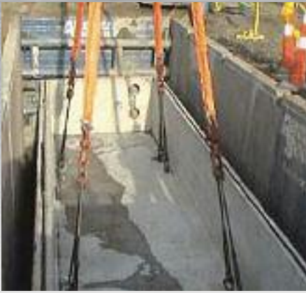
36' LONG HEAVY DUTY TRENCH BOX WITH AVENGER STYLE END CLOSURE PLATES
