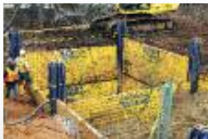
Remediation Slide Rail
